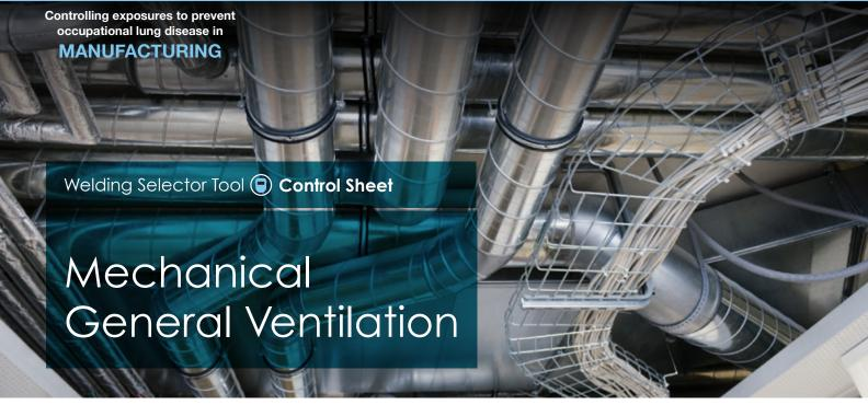
General ventilation is used to ventilate the room. Good general ventilation is needed to dilute fume generated from welding activities. Good general ventilation is not usually enough to stop workers breathing in welding fumes and, therefore, should be in place alongside local exhaust ventilation or respiratory protection.
