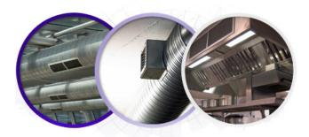
General (room) ventilation is used to ventilate the whole work area to dilute the fume generated from welding and stop it building up over the shift.
