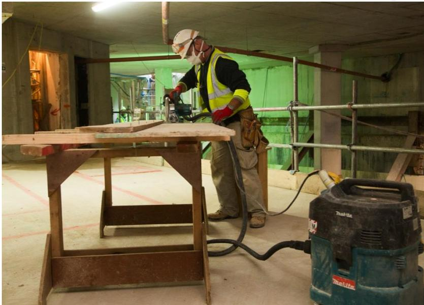
Where power tools are used on-site for wood working, dust exposure can be controlled by using local exhaust ventilation (LEV). Most commonly in construction this will involve on-tool dust extraction consisting of:
